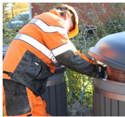
Picture 3.7 Remove the lifting loops.
