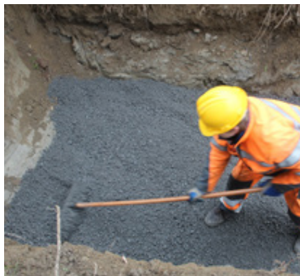
Image 3.1. 50 mm of 0-16 mm crushed gravel can be used for levelling.
