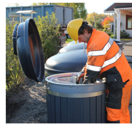
Picture 3.8 Open and straighten the lifting bag before placing it in the container.
