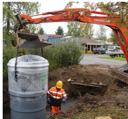
Image 3.3. Lift the container to the installation pit by using lifting loops. Make sure that the container is straight and level.
