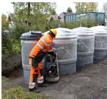
Image 3.5. Ballast material is then placed on top of the crushed stone (anchoring). Use a spirit level to ensure the container is straight and level.
