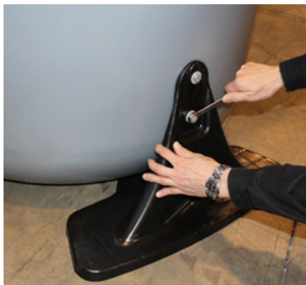
Image 3.2. Fix the plastic bottom anchors into the container using two bolts.
