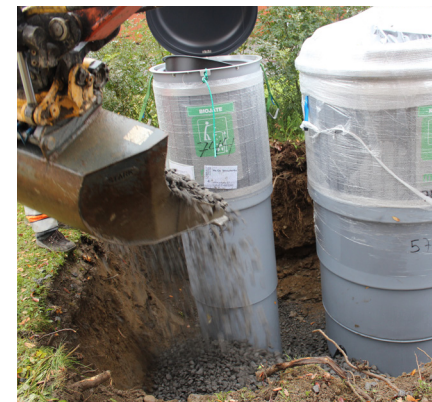
Image 3.4. Fill the installation pit using gravel 16-32 mm, ballast material and suitable finishing material.
