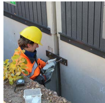
Figure 6. Tying the container bodies together
