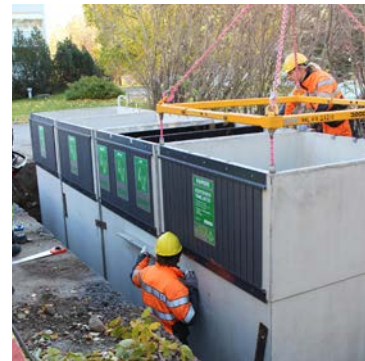
Figure 5. Checking the straightness
