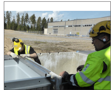
Image 9. Fastening the plastic well to the concrete well.
