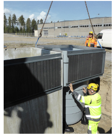
Image 8. Lifting the wells to the installation pit
