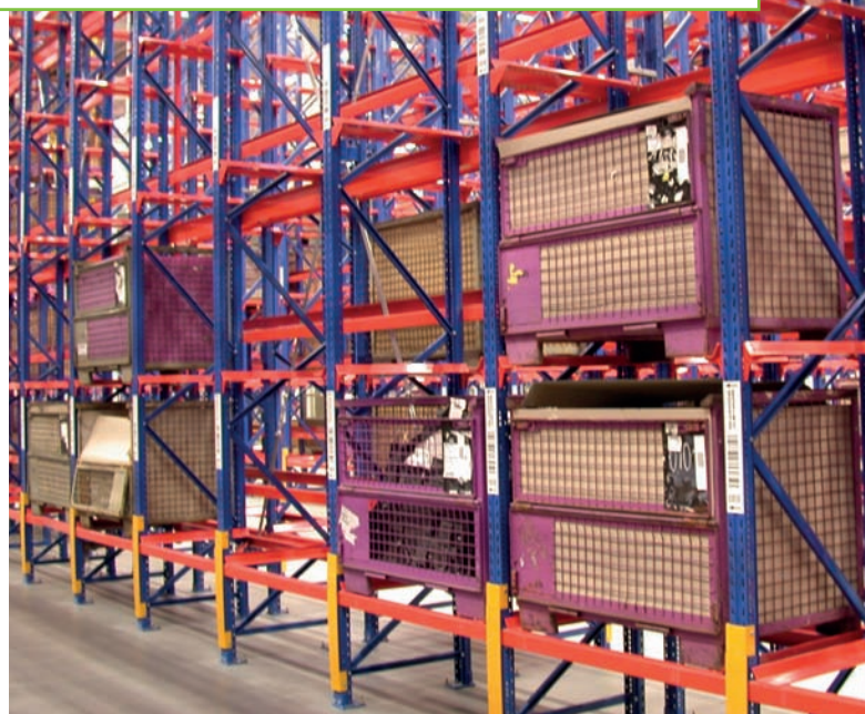
Open face racking
